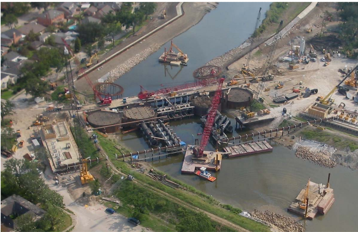
Orleans Avenue Outfall Canal Interim Closure structure under construction.
